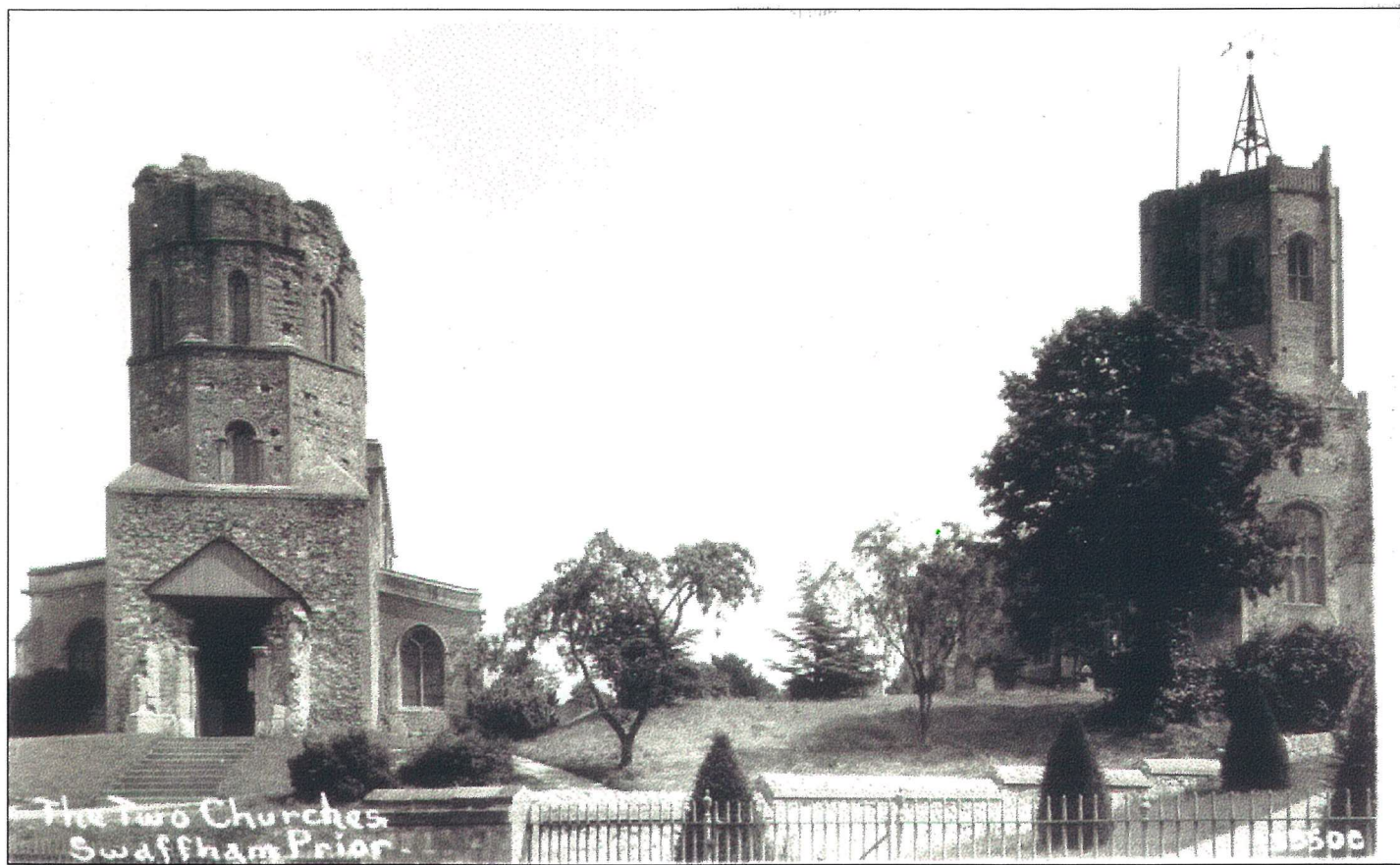
The Two Churches (Taken from the High Street)
