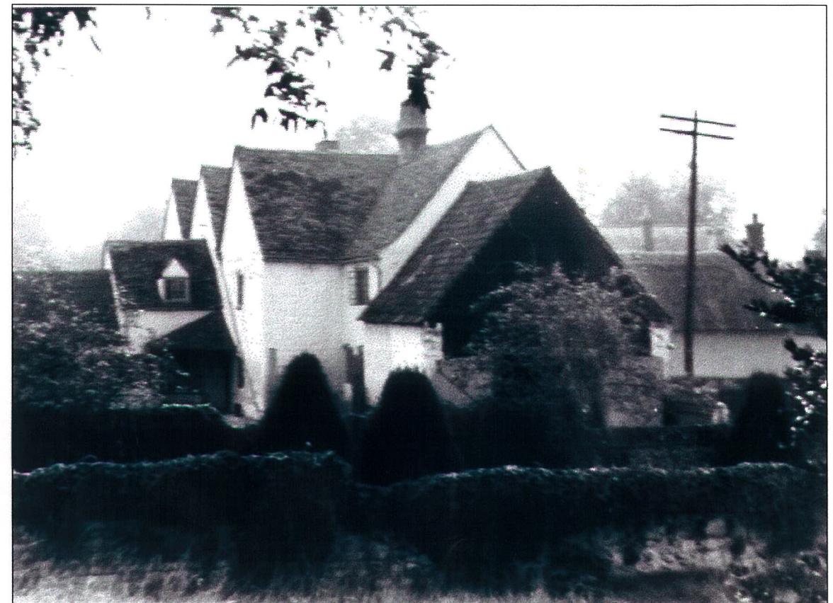
Anglesey House (Back view, taken from the churchyard)
