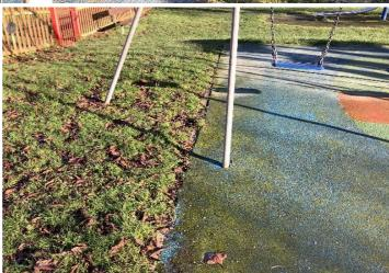
**Finding:** There are significant gaps (over 30mm) between the surface and the edging or between the joints in the surface; these are large enough for a small foot to enter
